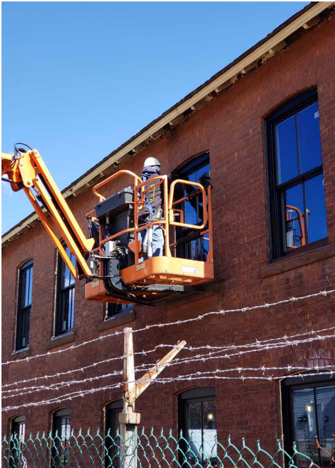
Construction at Swift Factory, Hartford, Connecticut
